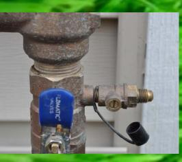
Step #5— Open the test port with a flat head screw driver. If no water comes out of the port, you have successfully turned off the water to the backflow prevention device. Close the test port and proceed to step #6. (some residual water may leak from this port, but it will stop) If water comes out of the test port and does not show signs of stopping, review the steps above. Proceed with the steps until step #5 is a success
