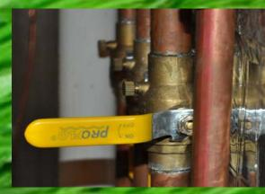
Step #3—Turn the shut off valve 90 degrees to the pipe as shown above. This will turn off the water to the backflow prevention device.
